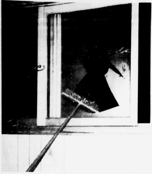
The above photos show only a fraction of the damage recently caused by young vandals to a building in Powder Hollow. The three-story, 8-foot-long wooden structure is used as a warehouse by Plasticoid Products. The building contains 44 windows, not
