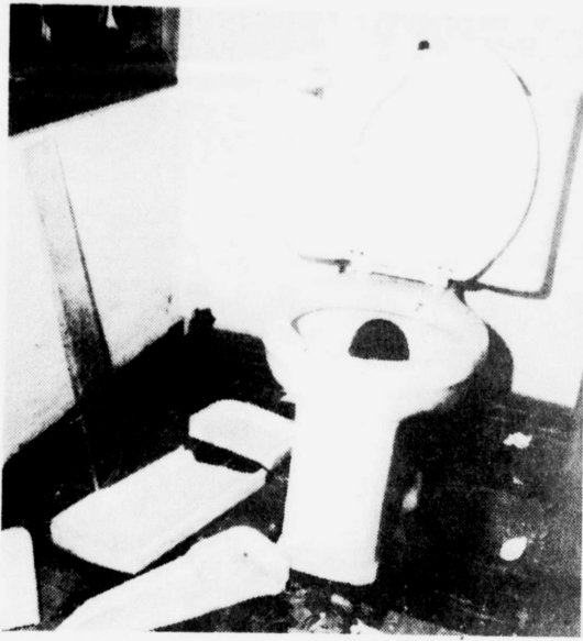
one of which escaped damage. Many of the windows were screened and boarded up but these did not deter the vandals. The wrecking crew did not confine their work from the outside, having also entered the building. The far left photo shows one of the instru-
