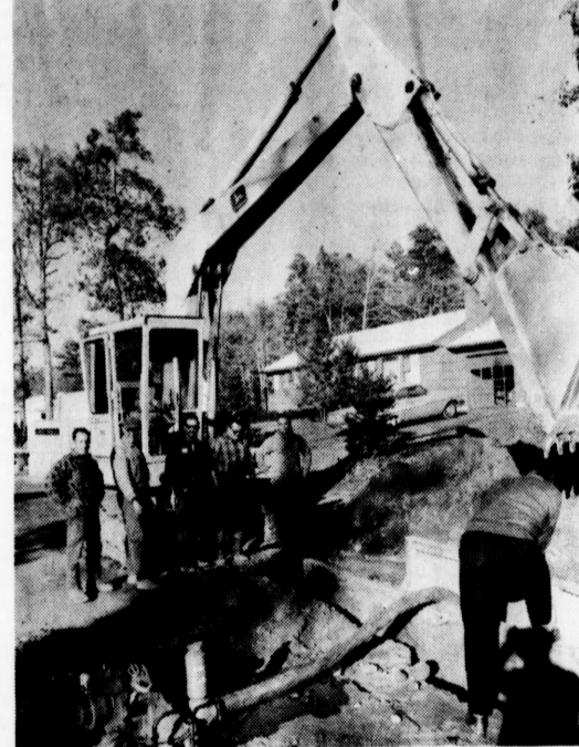
SEWER CONSTRUCTION, a $15 million project, is on a townwide basis.
