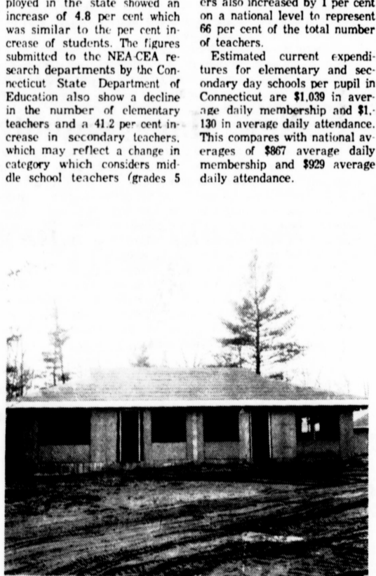
Woodside Park Pictured above is one of the double units of Woodside Park, an elderly housing project on Raffia Rd. The project features 40 units, consisting of 30 single and 10 double accommodations. Building is expected to be finished in May or June.
