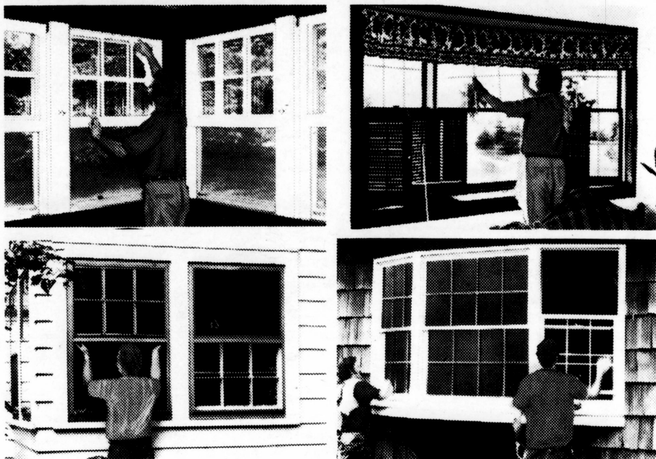
In window washing "derby" using professional housecleaners, Andersen windows with removable grilles and insulating glass (right top and bottom) took less time to clean (2½ hours for 30 windows) than multi-light windows with self-storing storm sash (left top and bottom). Latter took three hours for 15 windows. Time and work-saving were also reflected in lower cleaning costs.
