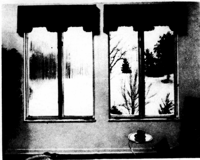
The single-glazed window (left) is subject to messy condensation caused by cold outside air striking a window warmed by indoor heat. The ponderosa pine window with insulating glass (right) stays clear and dry. Used with wood sash and weatherstripping, insulating glass keeps window temperature stable. This avoids the cause of condensation.
