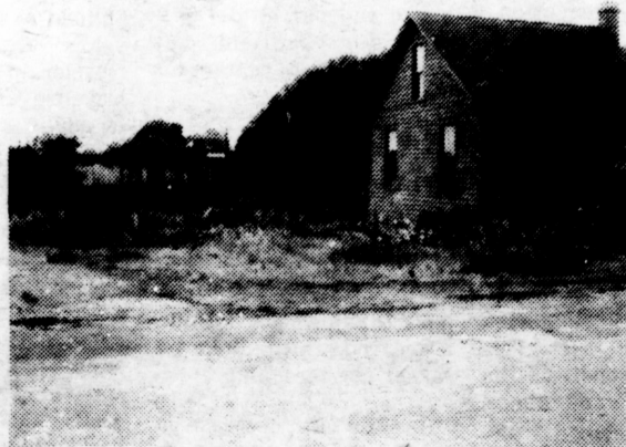
The Coal Smyth Coal Co., the remains of which are pictured served the Thompsonville area.
