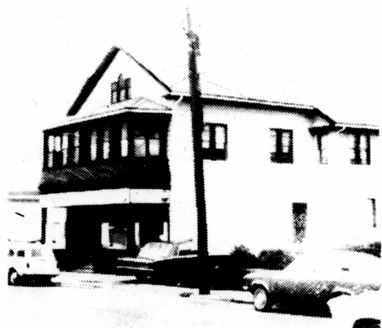
Prior to renovations the building pictured was the Methodist Church which served the Thompsonville area. Note the church-like proportions of the building and the three windows in the third floors.
